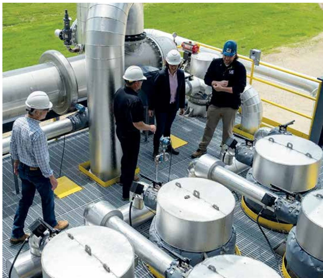
Aerial view of Whitefox ICE™ installation at United Ethanol in Wisconsin, US, 2019
